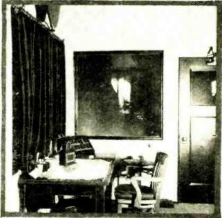
liere we have the microphone relay based in the announcer's booth; here the mirrophone control may be switched to studios or remete con-trols by pressing buttons; another button cuts the station off the air, in emergencies. Through the windows the announcer views the studios and the operator's control room illustrated on the opposite page. The elocability device is a new type of microphone. clock-like device is a new type of microphone.
