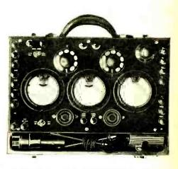
The Weston "Model 547 .4.C.-D.C." tester as it appears when the cover is removed. It both A.C. and D.C. screen-grid tubes. It tests
