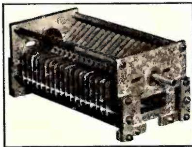
America, Micalex insulation is employed. Type R-39 insulation, a special development of the Radio Frequency Laboratories, can be supplied if desired in place of Micalex. The condensers are of variable capacities from 0.0005 to 0.00005 mmfd. Prices range from \$47.50 down to \$41.00
