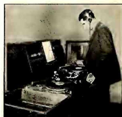
graph records for broadcast programs. The turntables are available in either single or double units operating at either 33 $\frac{1}{2}$  or 78 r.p.m. At the present time the equipment is in use at approximately twenty broadcasting stations. The equipment is not sold outright but is loaned to the station under a three-year license agreement which includes complete servicing by ERPI. The following stations have this equipment at the present time. In the following list
