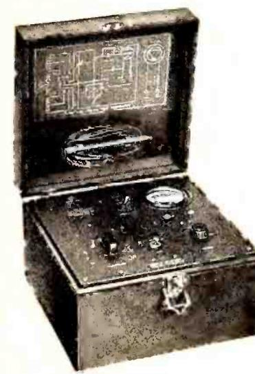
One of the new test oscillators for the radio service laboratory is now ready. It will deliver a modulated radio-frequency voltage at any point in the broadcast band (500 to 1500 kilocycles) and at 175 and 180 kilocycles. The tuning control is calibrated with an accuracy of 2 per cent.
