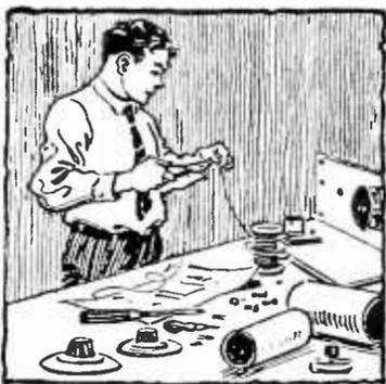
placing the honeycomb coil on the table beside the loop, or even by running the antenna lead-in past the loop within a few inches, sufficient coupling will be attained, when the antenna circuit is brought into resonance by tuning the variable condenser. However, I do not recommend that this apparatus be incorporated in the same cabinet with the set itself.
