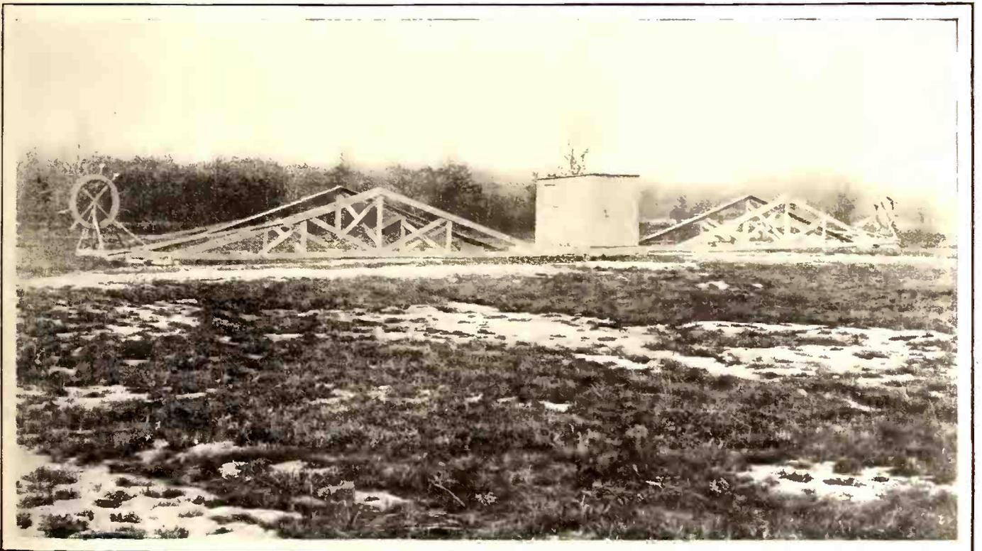
Figure 3. Two loops and receiver house where Friis' experiments were carried on
