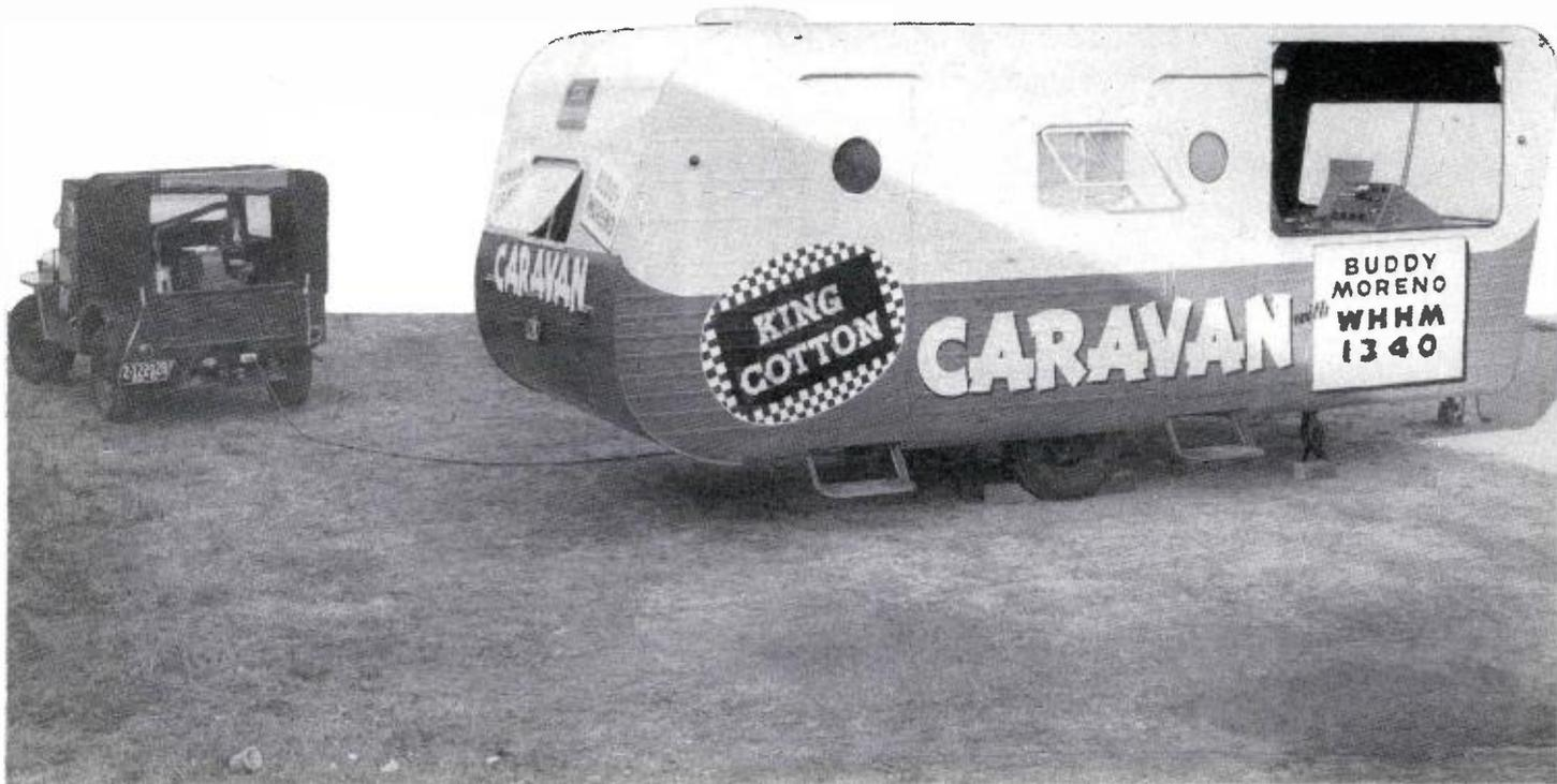
FIG. 11. Mobile studio connected to jeep-mounted power plant and ready for operation.
