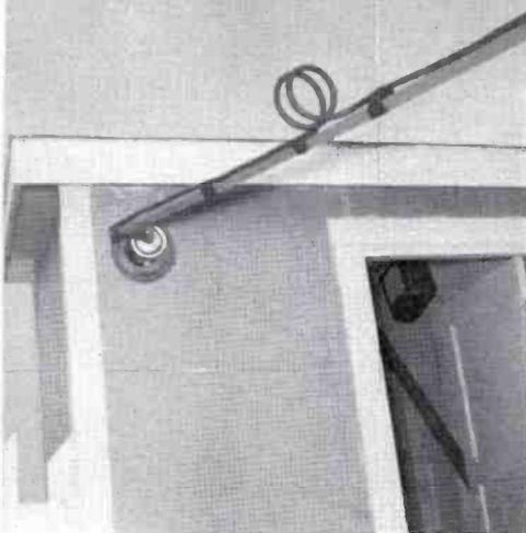
FIG. 12. Note two-turn coil formed in the antenna feed line to retard lightning.
