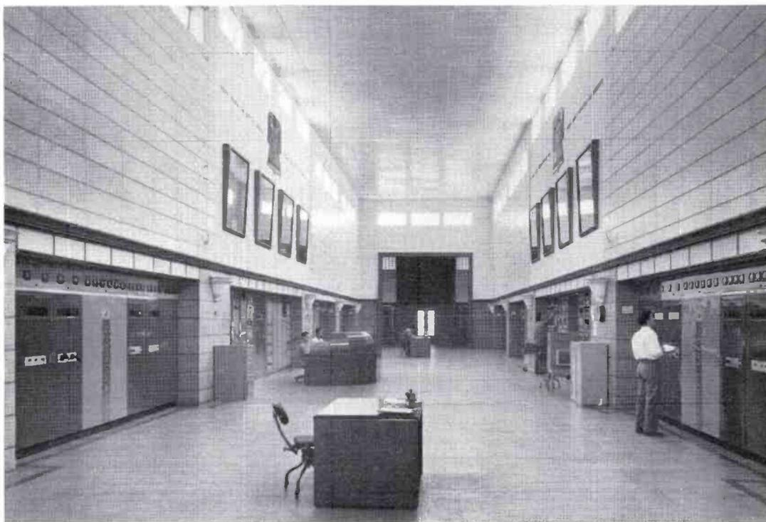
FIG. 39. Main transmitter hall at Gloria showing installation of eight RCA 50-KW Transmitters—four on each side.
