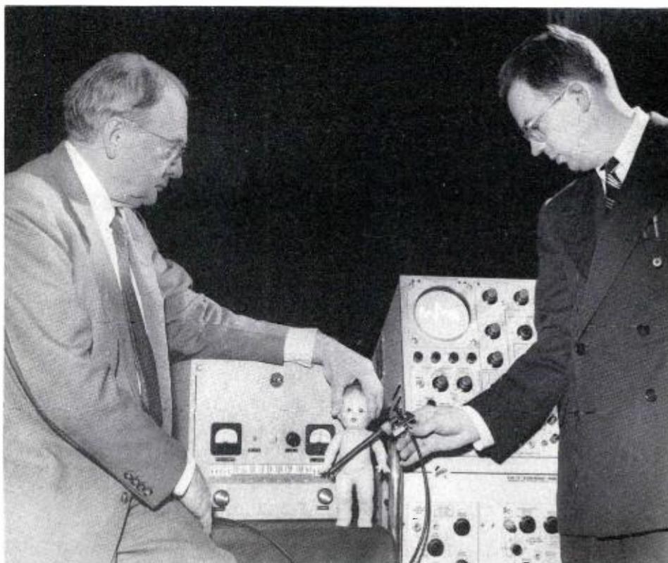
FIG. 3. Output of the "Radio Pill" is picked up by ferrite loop antenna held close to the body (doll in illustration). The antenna is connected to an FM receiver, and the output of the receiver is being fed to an oscilloscope. (The output could be fed to a recording galvanometer for making a permanent record.) The doctor can then observe the trace and diagnose the illness.
