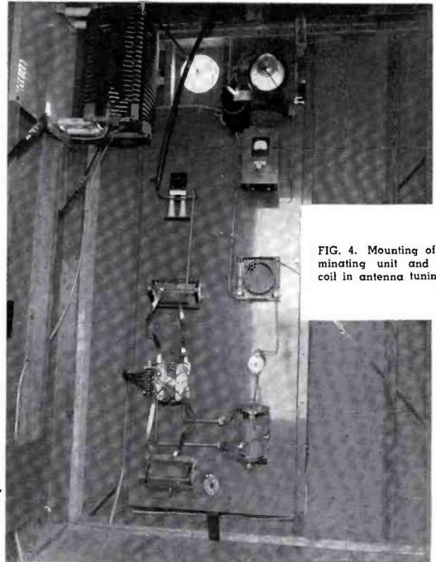
FIG. 4. Mounting of line terminating unit and isolation coil in antenna tuning house.
