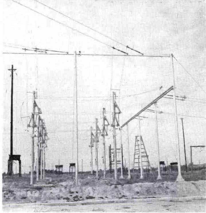
FIG. 51. Typical antenna switching group that handles two transmitters and four antennas.
