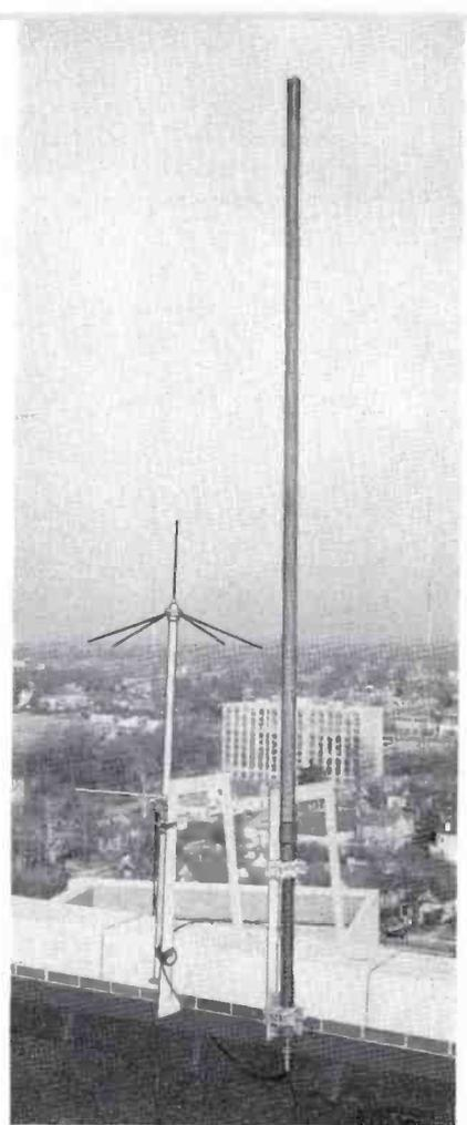
FIG. 5. The 150 mc and 450 mc receiving antennas mounted atop high building near WHHM studio.
