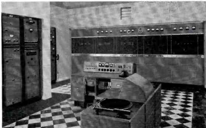
FIG. 5. Transmitter control room showing 1-KW auxiliary transmitter; speech racks and transmitter control desk. At left center, custom-built studio console with two 70-C turntables.
