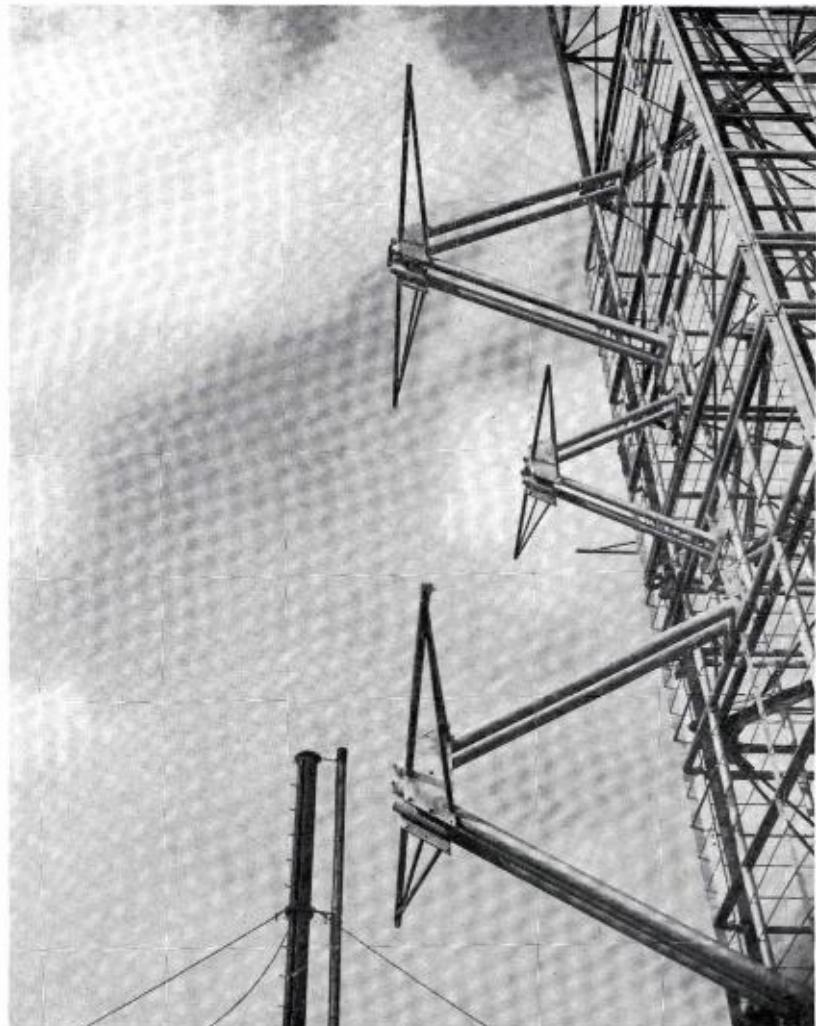
FIG. 14. FM Dipole Located in the Channel 2 Array.
