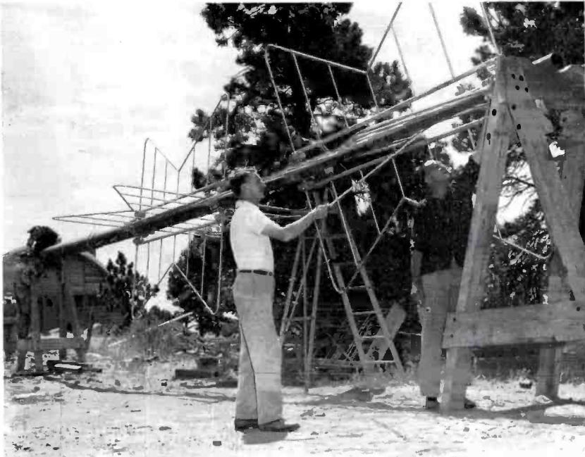
FIG. 1. Shown at the assembly of Superturnstile Antenna on Lookout Mountain are Tom G. Morrissey, Chief Engineer of KFEL-TV, and E. T. Griffith, Operations Coordinator of Broadcast Sales, Engineering Products, RCA.
