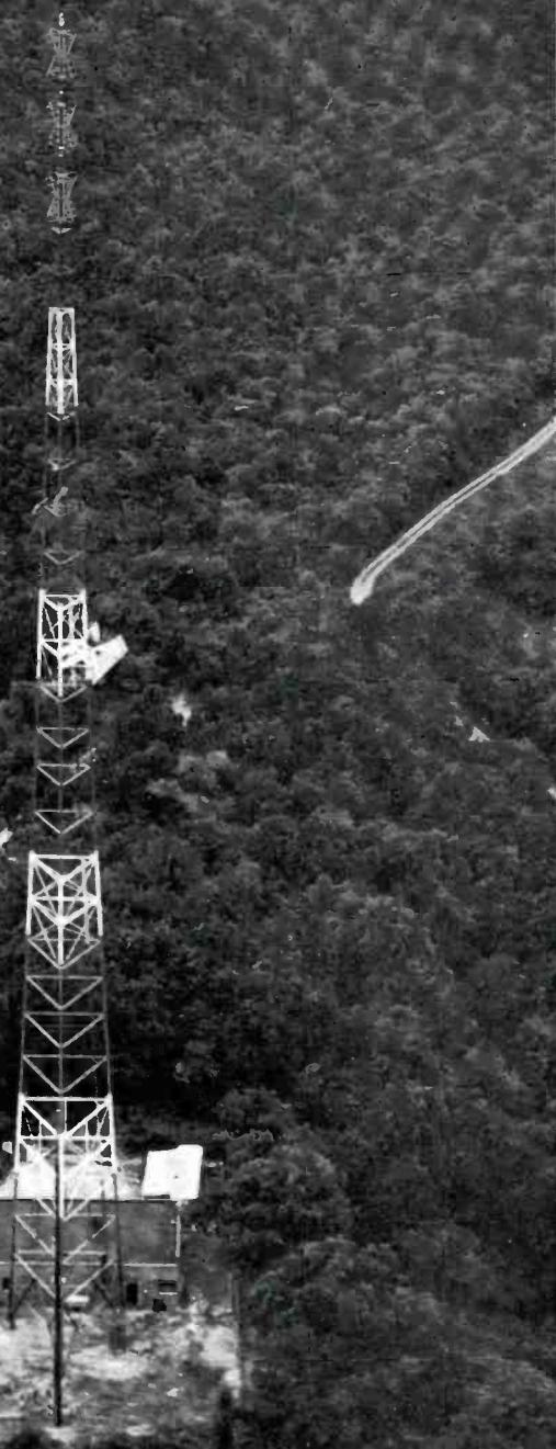
FIG. 1. WSAZ-TV tower with three-section Supertturnstile for Channel 3.
