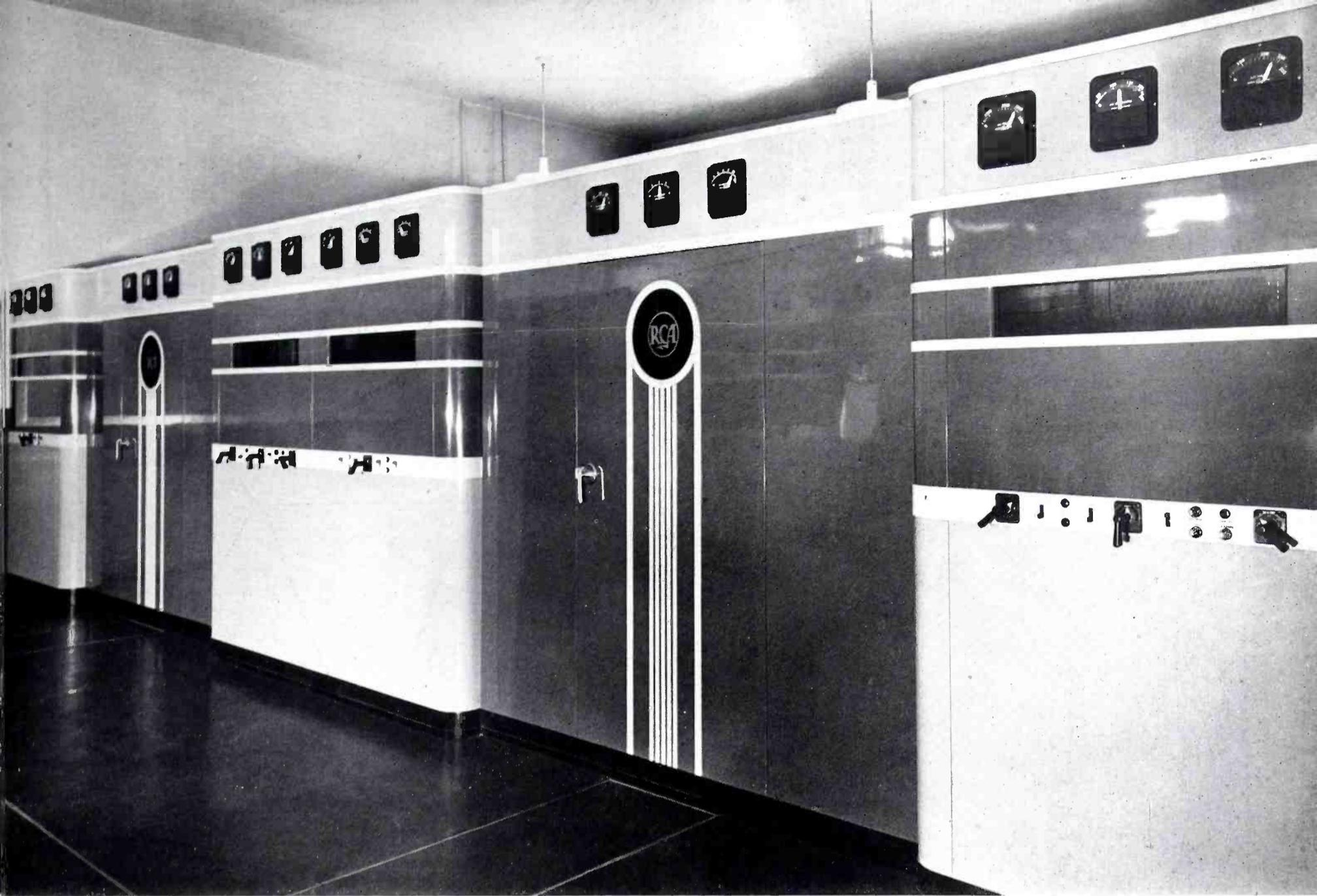
FIG. 4. General view of modulator-power supply panel arrangement. To place these units, as well as the r-f channels, within existing CBS building area required an alteration in the standard RCA enclosures and panels.
