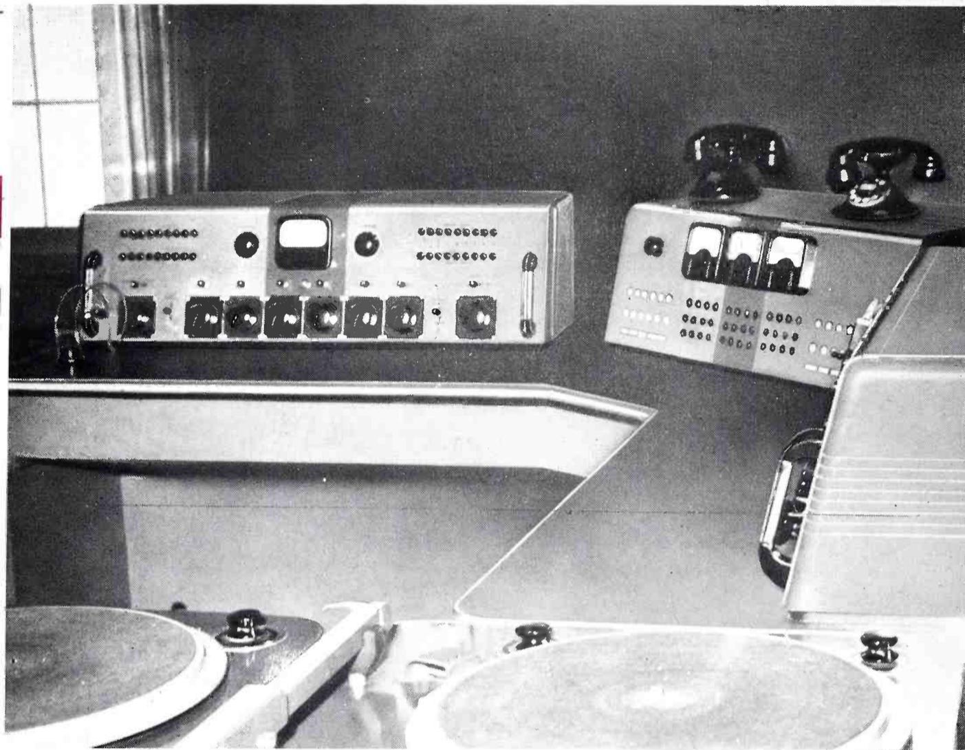
*Left*—The control room in the studios shared by FM station WSBF and AM station WSBT. Two RCA 76-B2 Consolettes handle the output of two studios. A master control console (center) provides monitoring and switching of outgoing lines to the two transmitters. The RCA 70-C Turntables may be seen in the foreground. In the studios RCA 41-BX Microphones are used.
