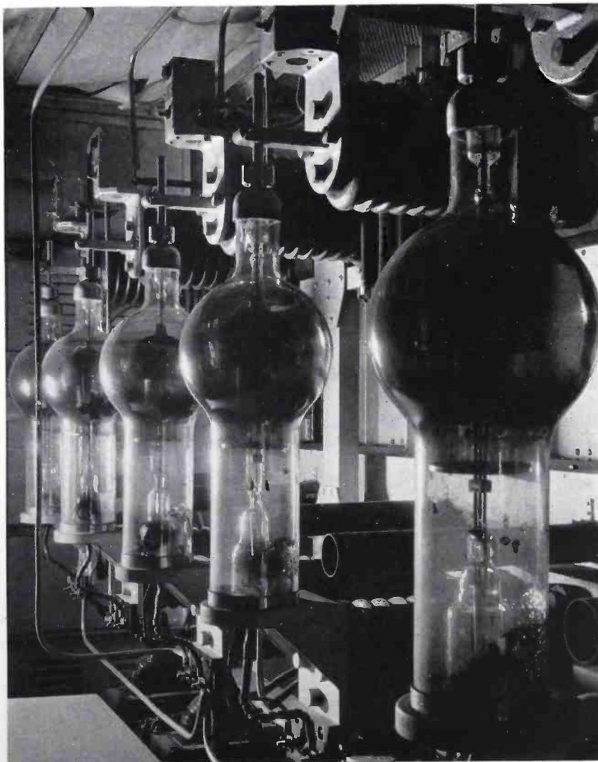
Lineup of rectifier tubes in the 50-C.
