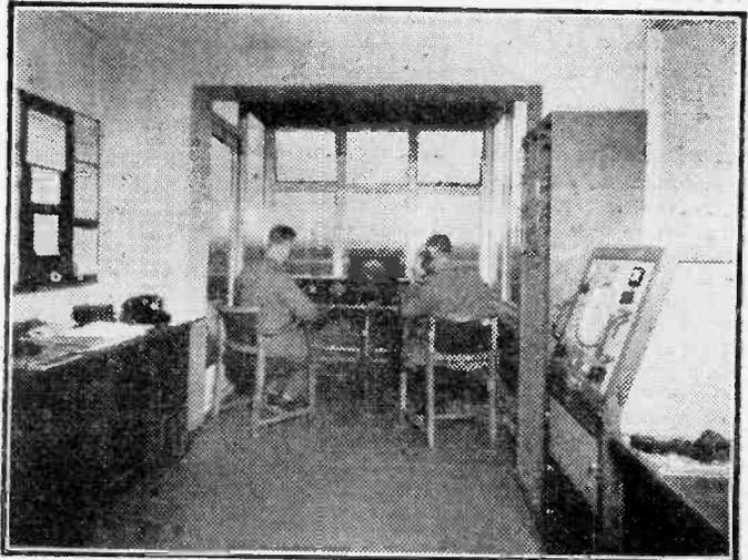
The Marconi AD.200 VHF/DF installation in the control tower at the de Havilland airfield, Hatfield. On the right can be seen the master control console and the twin receivers, and in the centre of the aircraft control officers' desk is a remote bearing indicator and twin loudspeaker.—See page 8.
