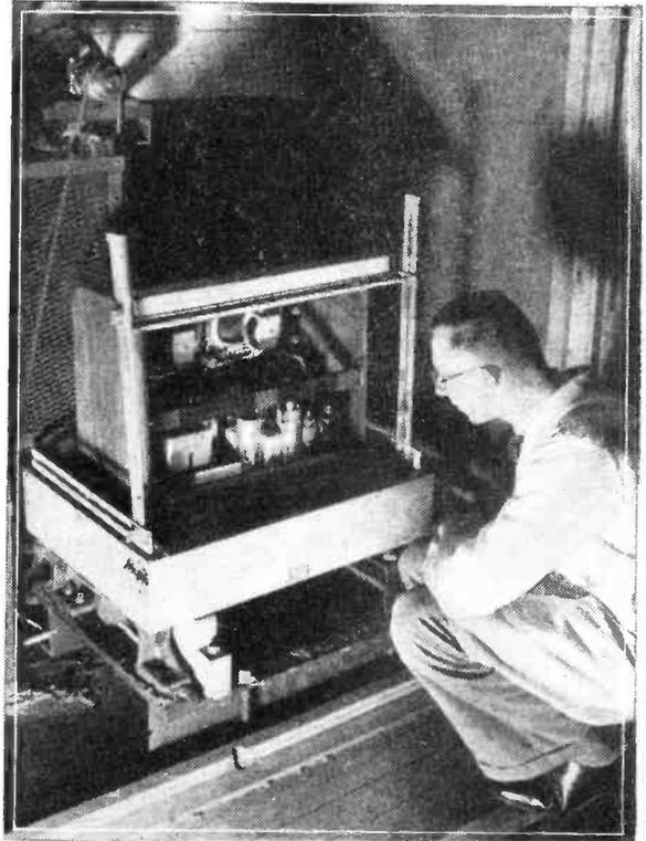
Every G.E.C. receiver gets the shock of its life on this machine. When the set has come through a gruelling test successfully it is judged O.K. for service overseas.
