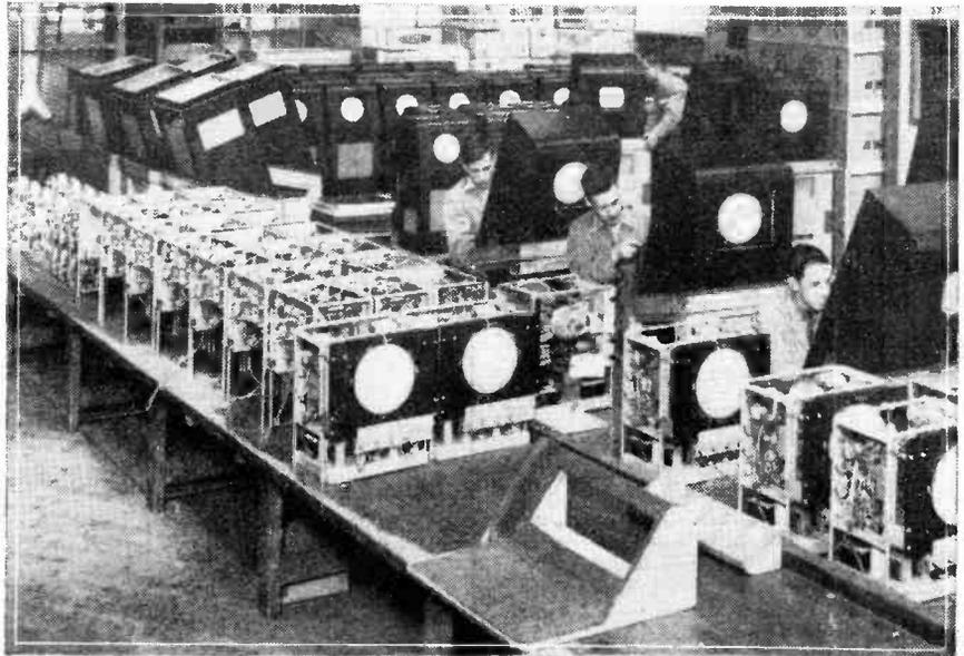
A typical view of the television benches in a modern radio factory, where final adjustments are being made to mass-produced television receivers.
