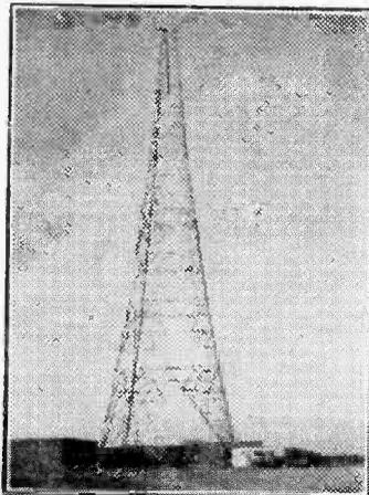
The aerial mast at Lichfield as it appeared when we went to press. The Marconi 16-stack aerial array is the first of its type to be designed and produced in this country.
