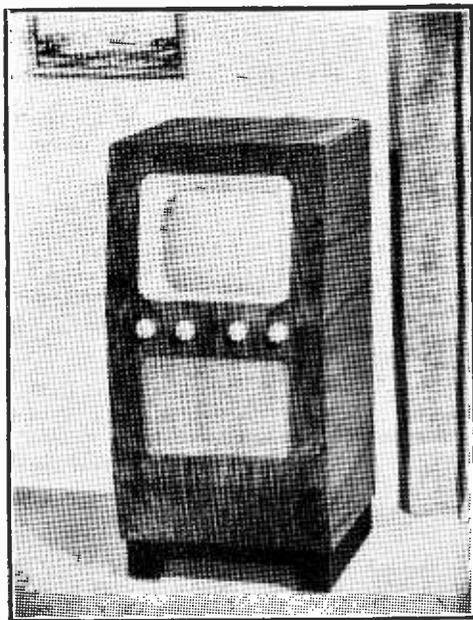
Pilot model CV34 with 12in. tube.
