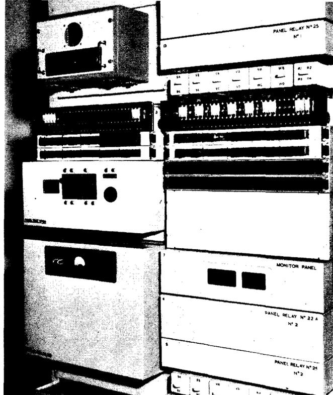
Fig. 5. G.P.O. Land-line terminal equipment. The W/T Distress Frequency Receiver is seen at top left and below it, the Auto-Alarm Equipment and associated Test Panel
