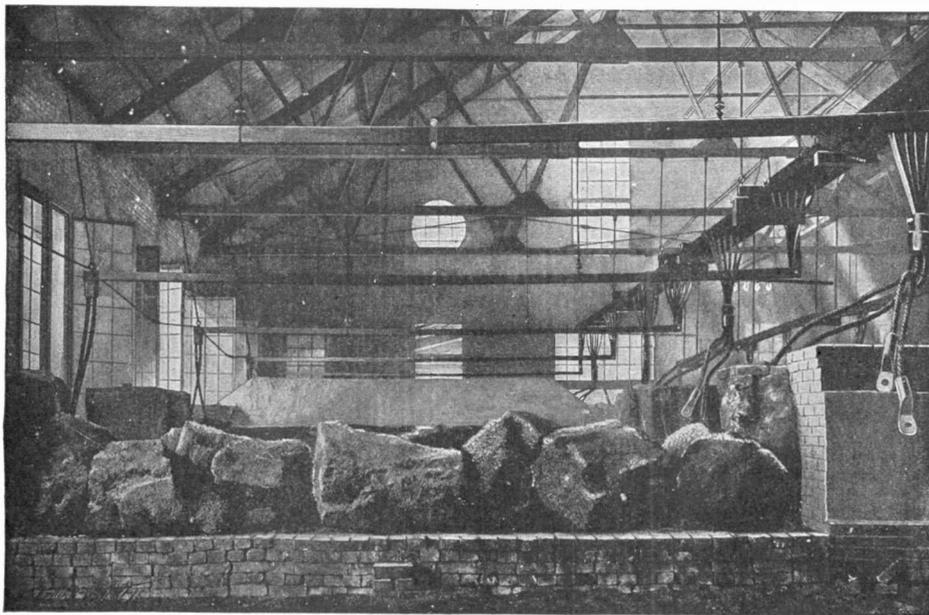
CARBORUNDUM FURNACE AFTER BURNING, SHOWING CRYSTAL MASSES
