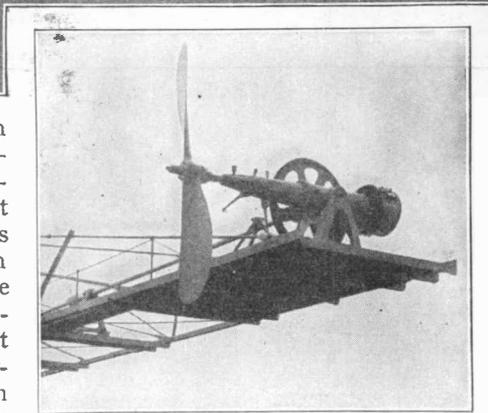
SWINGING CANTILEVER FOR TESTING PROPELLERS
