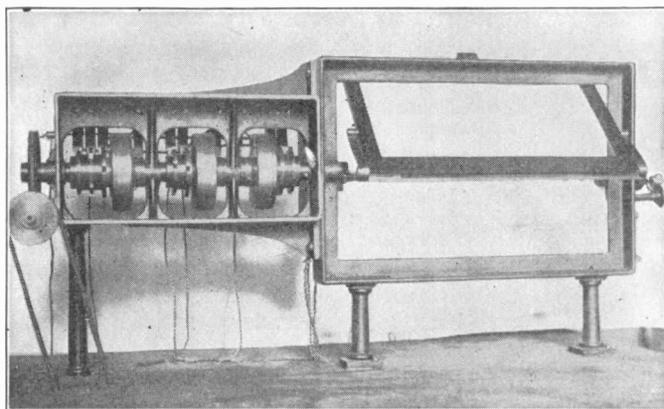
COPY HOLDER USED WITH CHECK RECORDING CAMERA
