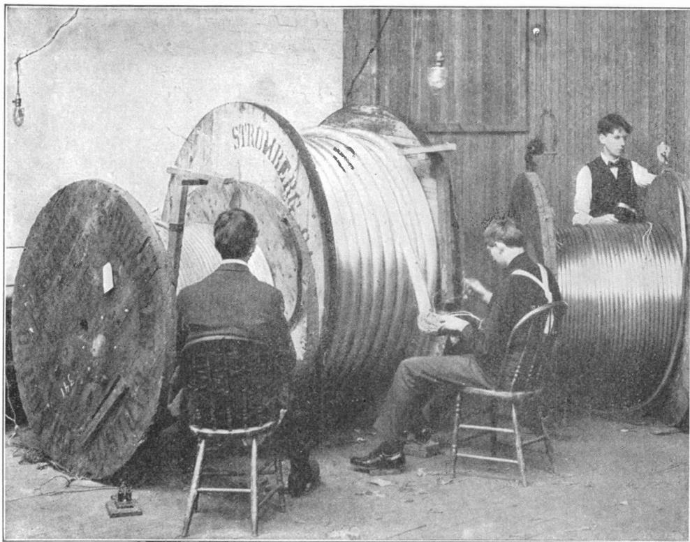
FIG. 6. TESTING CABLE. THESE MEN MAKE THE CONNECTIONS AT THE ENDS OF THE STRANDS
