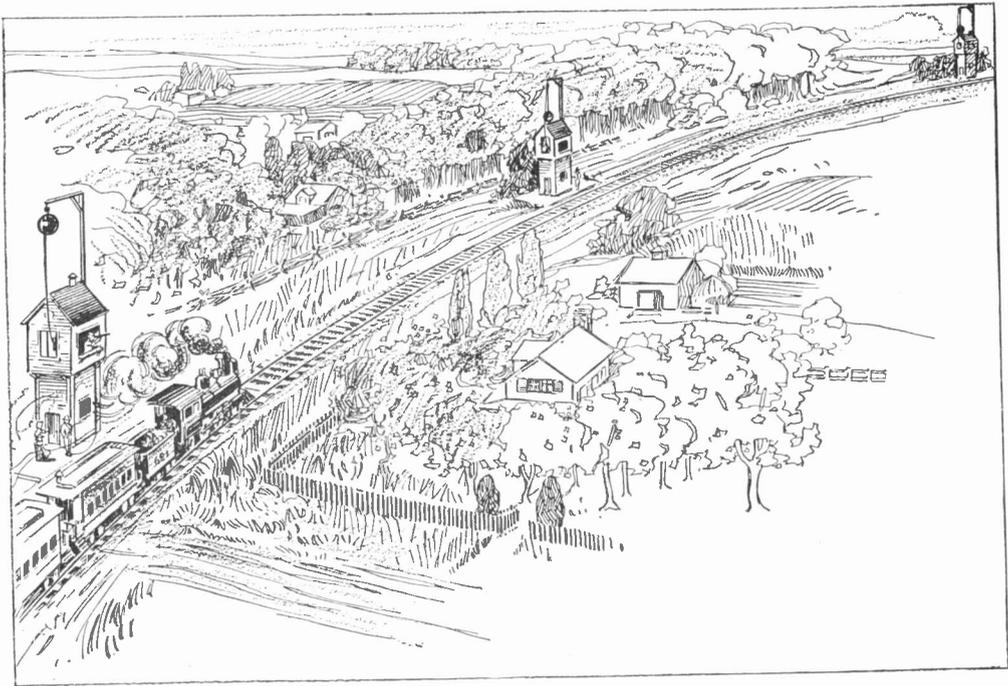
THE FIRST BLOCK AND SIGNAL SYSTEM AS USED IN ENGLAND
