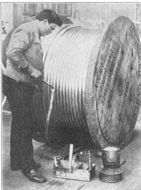
FIG. 7. SEALING UP THE END OF A TELEPHONE CABLE
