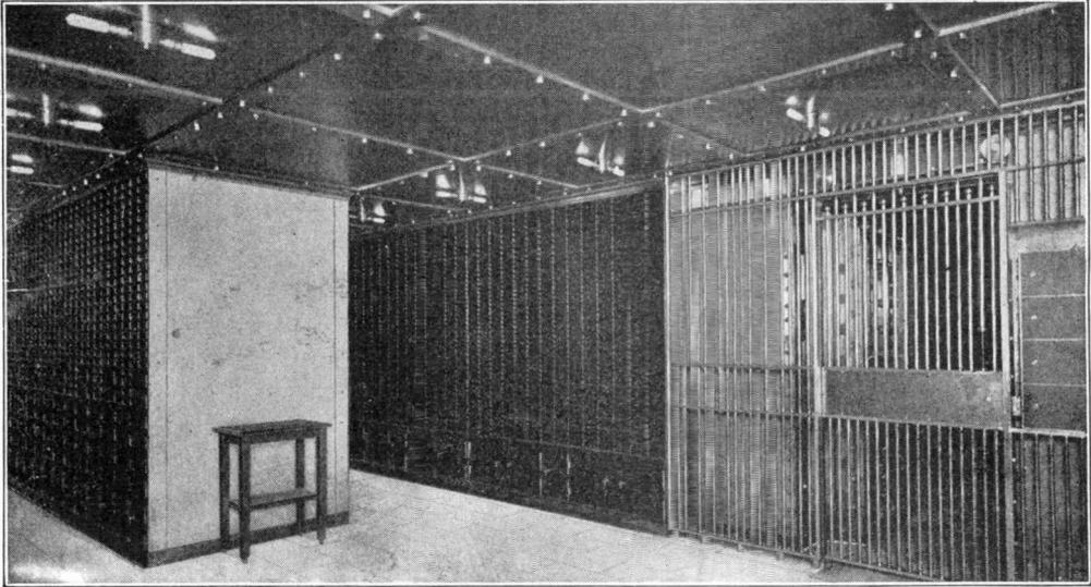
BANK VAULTS WHICH ARE PROTECTED BY A CHARGED WIRE MESHWORK
