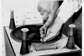
Fig. 2. Because speaker board is fixed by caulking compound, it is necessary to front-mount woofer. Staple or tack grille cloth over speaker cone to protect it against dust and pets.
