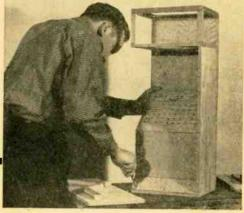
Side view of enclosure, showing its perforated resistive panel. All joints are screwed and glued.
