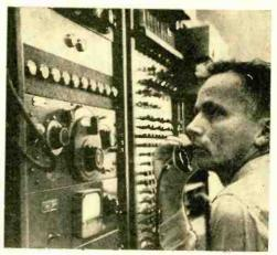
that determined which of ten numbers from 1 through 0 had been spoken into an ordinary telephone. It responded by flashing an appropriate light, as can be seen in the photo. At the time that the development of this device was announced, the Bell Labs people hoped to use it in conjunction with their telephone dialing operations.
