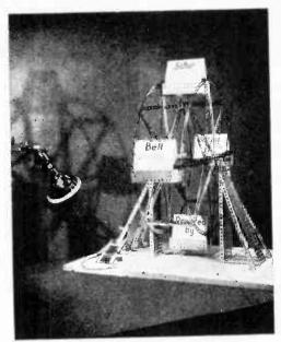
A toy ferris wheel which receives its power from light falling on a tiny piece of silicon. It was used to demonstrate principle.
