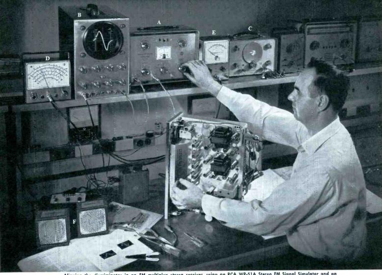
Aligning the discriminator in an FM multiplex stereo receiver, using an RCA WR-51A Stereo FM Signal Simulator and an RCA WO-91A Oscilloscope. Display on scope screen is the trace obtained at the output of a properly aligned discriminator.
