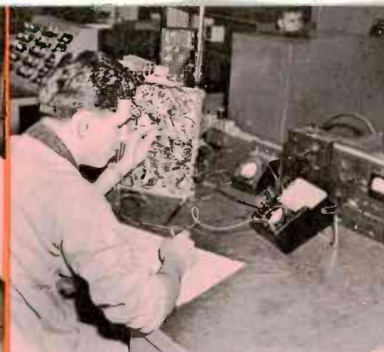
Voltage analysis is performed on the receiver, using typical equipment employed by Service Technicians. Resistance values are also taken here, and in the case of a TV receiver a sketch is made of tube placement.
