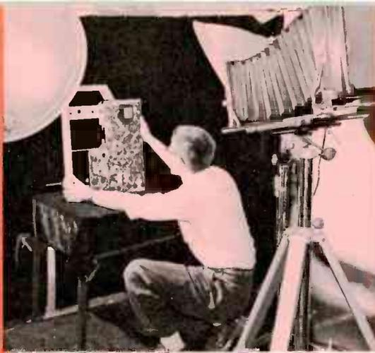
Next, chassis photographs are taken for complete parts identification; separate photos are taken of tuner, major sub-assemblies or complex design portions. A photograph is also taken of the equipment for identification.
