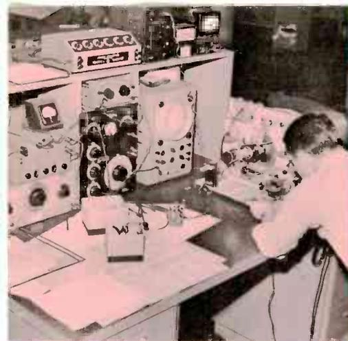
Continuing the analysis process, the receiver progresses through 13 separate operations: Data is gathered and recorded on controls, resistors, RF and IF components, transformers, chokes, speakers, deflection components, tubes and other parts.
