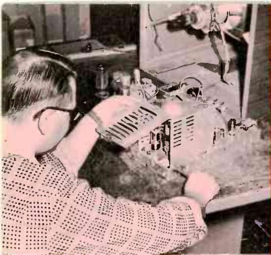
The first step in the processing operation is to remove the chassis from its cabinet. Notes are made on any unusual problems encountered; these are covered in the finished PHOTOFACT Folder.
