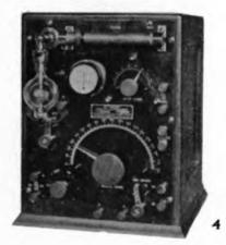
Fig. 1 illustrates Appearance of new De Forest Wireless Telephone and Telegraph Set for Portable Work.
