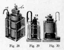
in Figs. 28, 29, 30 give only about onehalf to one ampere, while a battery as shown in Fig. 30 on account of the large surface of both zinc and carbon gives from 12 to 25 amperes, all depending on the size of the elements.
