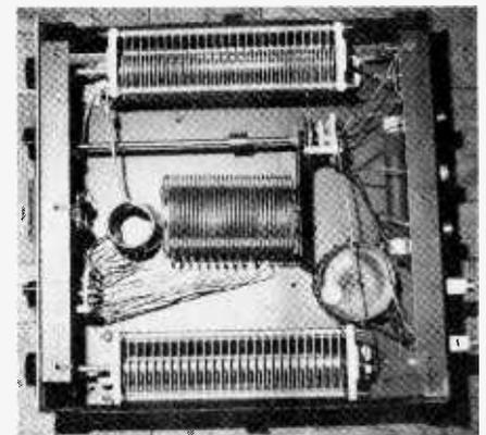
This inside view of the Versa Tuner IV shows rugged coils that let unit take 2KW.
