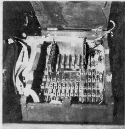
A special housing had to be built under the Cadillac's front seat to hold the Central Processing Unit and two disk drives of the Apple II microcomputer. The design of the Apple II allowed for its mounting in an unventilated area of the Caddy.
