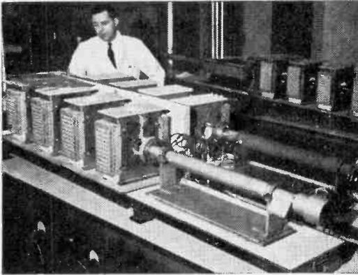
**ZONE REFINING** furnace is what this device is called. It's used for purifying Germanium in producing transistors. Selected blanks are heat-treated.
