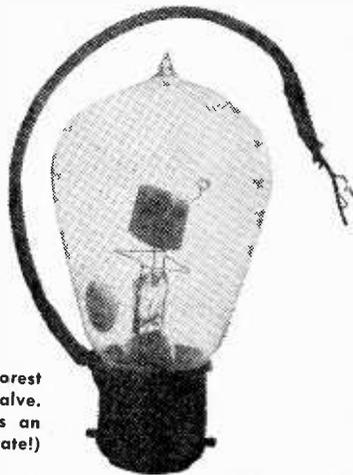
KID BROTHER to the DeForest Audion is this Fleming Valve. This two-element tube was an early diode . . . (Not solid state!)
