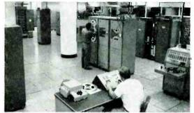
Four of the twenty-four Ampex FR-100 Tape Transports at the General Electric Missile and Ordnance Systems Department facility in Philadelphia.
