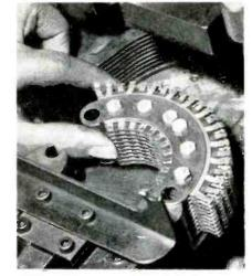
STEP 4—Removing sheared bank assembly from press after removing pins
