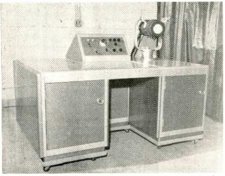
Self-contained console of playback unit, designed primarily as a master station from which a number of remote indicators can be controlled, is used as a training station, since it is provided with a complete operating indicator
