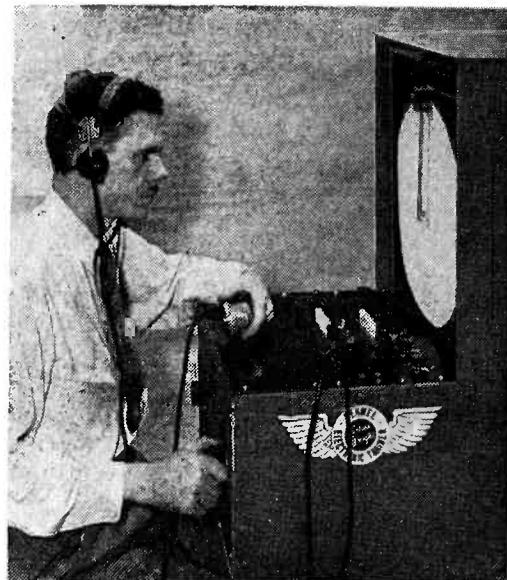
Flight-path recorder and automatic radio range of the Curtiss-Wright Dehmel electronic flight trainer for embryonic pilots
