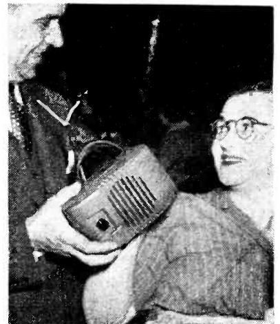
volume control and coiled cord has been designed. The speaker can be hung in any convenient place in the car after it has been removed from its outdoor shelf by the patron himself.
