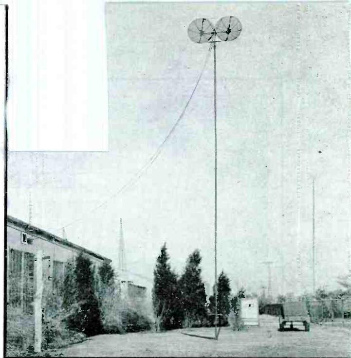
Antenna of the TRC-5 consists of two dipoles with parabolic reflectors atop a guyed fifty-foot pipe
