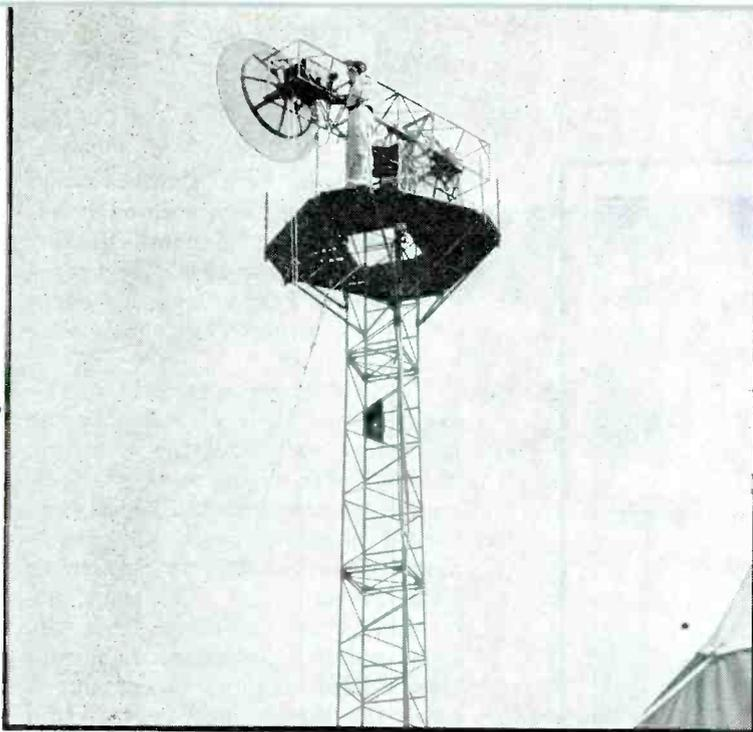
Transmitter and receiver of TRC-6 are mounted at antennas so that super high frequency circuits will be short
