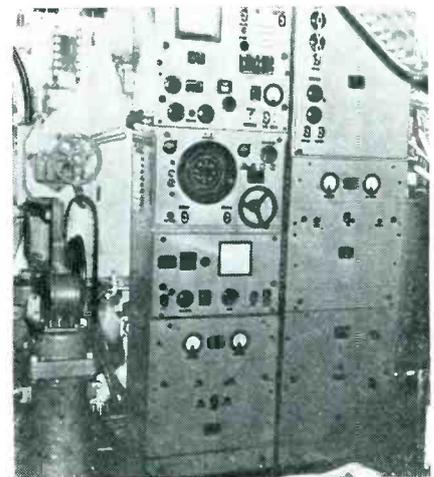
Modern echo-ranging sonar installation in a U. S. submarine. Right-hand rack generates supersonic voltages that energize the transducer which is lowered through keel of submarine by hoist mechanism at extreme left. Left-hand rack contains echo amplifier, target range and bearing indicators, and training control wheel
