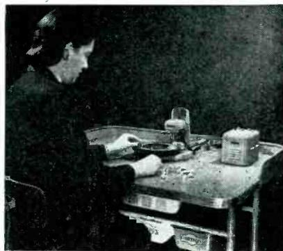
places each piece in the proper bin. The range of measurement possible is between 0.0001 and 0.03 inch. Contact spindle pressure is adjustable from 4 ounces to 1 pound.
