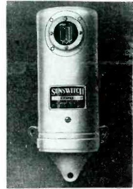
nightfall. The unit consists of conventional electron tubes, a photoelectric cell and relay. Overall dimensions are  $9\frac{1}{2}$  x  $4\frac{1}{2}$  in. diameter. The weight is  $4\frac{1}{2}$  pounds.
