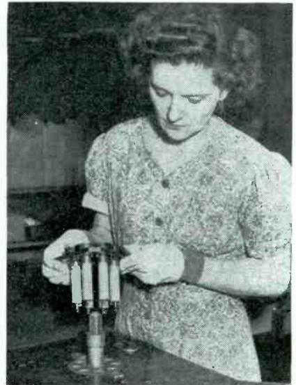
Eight elements for test equipment gear are assembled with a preformed ring of solder in position at the juncture to be sealed, then secured in a fixture. The operator lowers them through the holes into the field of an induction coil connected to a 15-kw RCA r-f generator used in the Camden plant of RCA Victor Division
