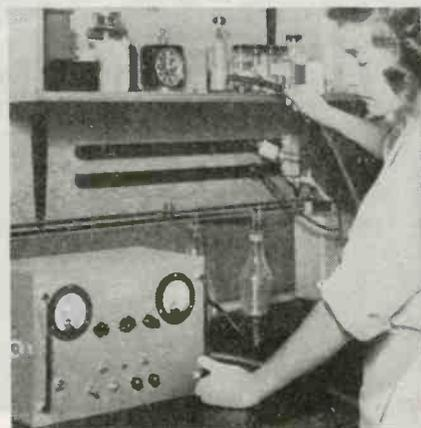
Instantaneous detection of mercury vapor in the air of industrial plants is made with this G-E instrument. It measures concentrations as small as one part in 200,000,000
