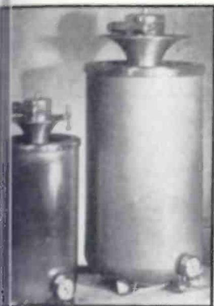
Two sizes of Lapp Insulator Co. precision capacitors show aluminum shells, gear head drives, and indicator pressure gauges. Also featured are adjustable provisions for external flash-over.
