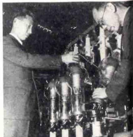
Two engineers from the Chinese Central Broadcasting Administration fit tubes into the rectifier unit of a high-power broadcast transmitter recently built in Great Britain for China
