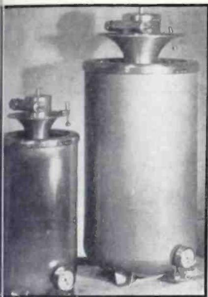
Two sizes of Lapp Insulator Co. pressurized capacitors show aluminum shells, gear head drives, and indicator pressure gages. Also featured are adjustable provisions for external flash-over
