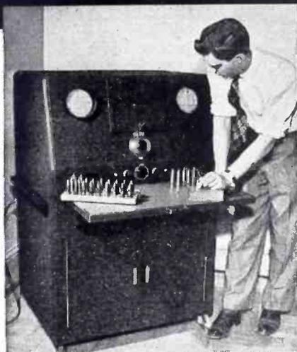
GOOD bad GOOD GOOD bad... 6,500,000 bullets, rejected because of a mix-up in copper cladding measurements, were re-sorted by the DuMont Cyclograph... 99% of them salvaged!
