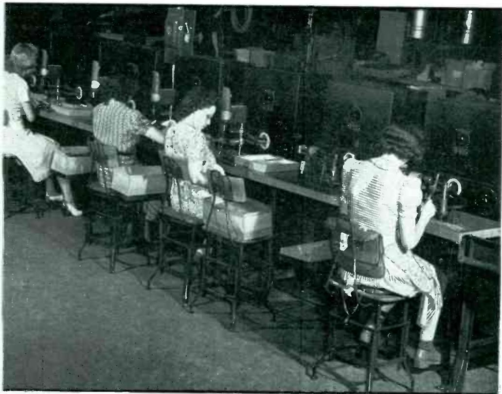
Fig. 4A—Installation of spot-welding controls operating bench-welders
