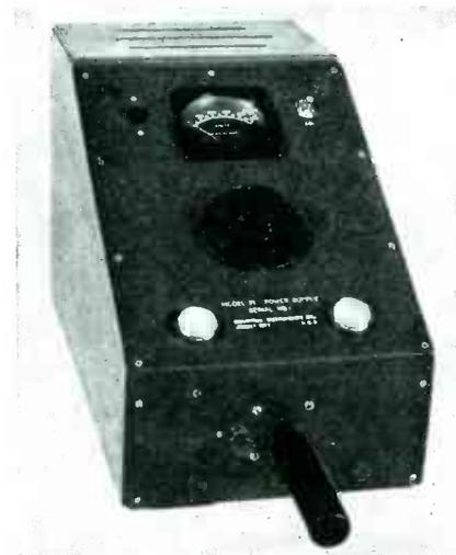
d.c. A self-incorporated safety switch makes the power supply inoperative if chassis is removed from case or otherwise disturbed.
