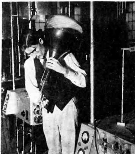
Removing the soot which was left after annealing to prevent too rapid cooling and guard against cracking
