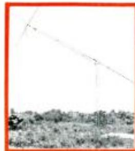
**Fold-over** The No. 25, as well as heavy-duty No. 40 communication tower, can be converted into "fold-over" towers for amateur use . . . the only tower of its kind. They let you work "on the ground!"
