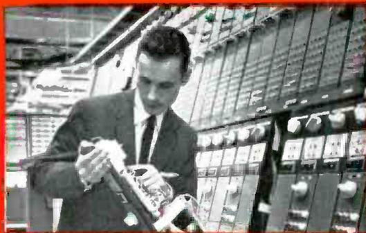
Checking panel wiring of Simplex console
