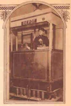
When a subject is to be examined for the position of a motorman on a trolley car, where quickness of thought and instant deter-mination are an important factor, he is placed in a realistic reproduction of the front end of such a car as illustrated above. An observer seated directly to the rear records all movements and reactions.
