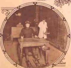
The reflexes of an automo-bile or 'bus driver are tested by psycho-galvanic apparatus as illustrated at the left. The response of the candidate to various suggestions is recorded and measured. The rear of the observation board connected to the device illustrated at the left is shown at the right. The observer has instruments directly in front of him which indicate and accurately measure move-ments of the subject.
