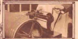
At the extreme left is shown another test for motormen. Here the driver is placed on a platform and a motion picture proj-ected on a screen in front of him detailing the incidents along a route. The candi-date's reactions to the various illustrations are noted. The photo at the left shows the Benet oscillograph for measuring the speed of motor nerve impulses in the hand and arm. arm.
