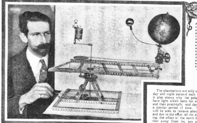
the left shown the completed model of a planetarium, a machine which exhibits clearly the motion of the earth and the moon and the or-bits of both of these bodies about the sun. It also shows the different positions of the earth in summer and winter.
