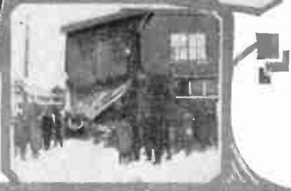
Above: The original photograph and reproduction after being transmitted by radio. The top photograph is the original and the bottom one the reproduction. At the receiving end, no trace of the screen used in making the half-tone is visible, the only effect being a few vertical lines.
