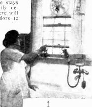
THE long cord connects to a reversing switch for the motor.
