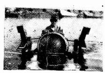
A ten-year-old boy is shown seated in one of these paddle-wheel boats. They are operated by turning the cranks by hand and steered by warying the speed of the two paddle wheels.
