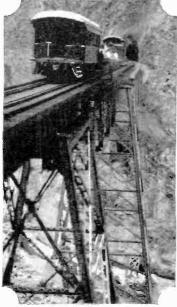
As the safest mountain railway in the world the Peruvian Railway uses no curves or horseshoe turns. Visco Switchback, shown above, pictures the construction needed to obtain altitude.
