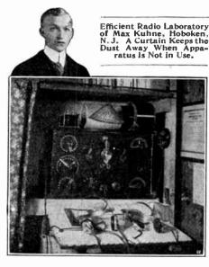
ser, audion detector with set of high vol-tage batteries and rheostat, and a pair of E.I. Co. 3,000 ohm 'phones. All instru-ments are mounted inside of the cabinet controlled by two hard rubber knobs.
