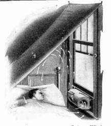
Indirect Drait, Electrically Driven Window Ventilator.
