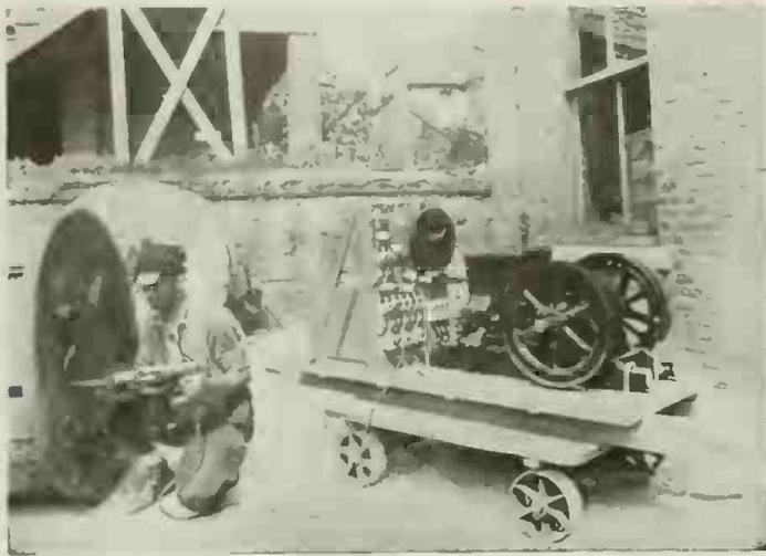
Extremely Compact and Efficient Portable Engine and Dynamo Set for Supplying Current to Electric Hammers and Drills, One of Which is Here Shown in Use.
