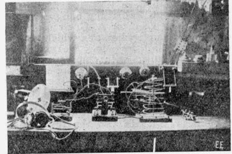
Here is a description: Sending, one-half inch coil; test tube condenser; helix; spark gap and key. I run the coil on a step-down transformer and it gives a little more than a 1/2-inch spark.
