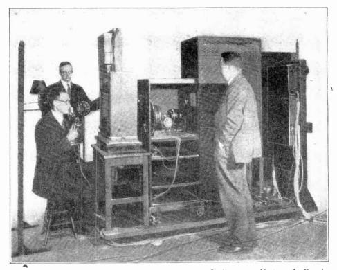
Fig. 98. A subject sitting before the transmitting mechanism. In the center cabinet are the 60-cycle and 2,000-cycle A.C. motors which drive the perforated disk. The light from an arc in the cabinet at the rear passes through the holes in the revolving perforated disk and falls on the face of the subject. [Photos courtesy of Bell Telephone Laboratories.
