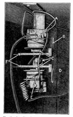
Fig. 81. A, coil producing alternating current of ten cyc'es; B, mirror; C, permanent magnetic circuit; D, frame; E, receiving coil of the tuning fork connected to the triode tubes; F, legs of the tuning fork (oscillating armature of the alternator).
