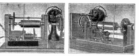
11. On the left is the transmitting apparatus for the transmission of pictures by radio. The coil and gap may be seen fixed on the base supporting the whole set. On the right is the receiver with the coherer and writing device mounted on the electro-magnet armature. Fig. 31.
