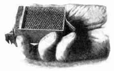
Fig. 89. The cellular structure of the image-projection tubes used in Baird's television apparatus.
