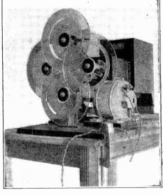
Fig. 44—Left. Mr. C. F. Jenkins and his apparatus for the transmission and reception of photographs by radio. This apparatus copies half-tone camera studies from flat surfaces, transmits them, and at the receiving end they are impressed on common photographic plates.
