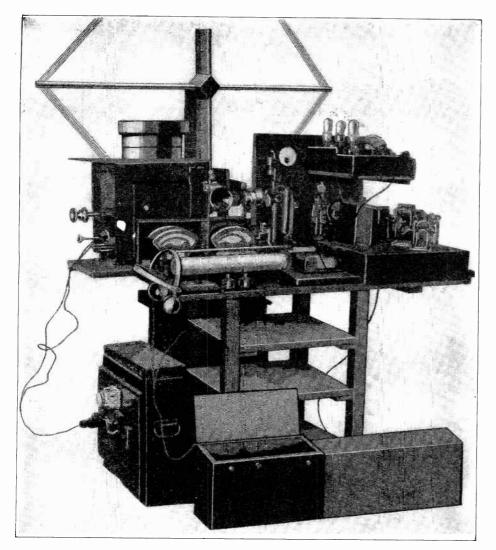
Fig. 43. The Mihaly Telehor machine. I is the arc lamp, 2 the light relay oscillograph, 3 the tuning fork, 4 the screen, 5 the diaphragm, 6 the escillograph, 7 electro-magnet of phonic drum, and 8 the brush.
