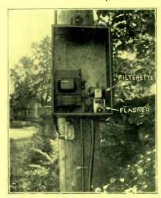
Fig. 3. Photograph Showing Installation of Filterette FS-110 in a Typical Traffic Flasher Control Box.
