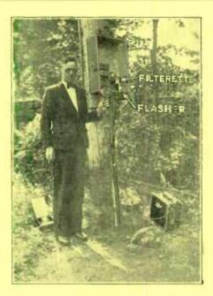
Fig. 1. Massachusetts State Highway Engineer Checking Interference from a Traffic Flasher
