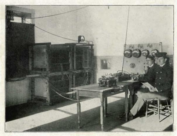
STATION AT CLEVELAND, OHIO, CLARK WIRELESS TELEGRAPH Capacity 10 K. W. This station has been in operation three years and has been improved every year
