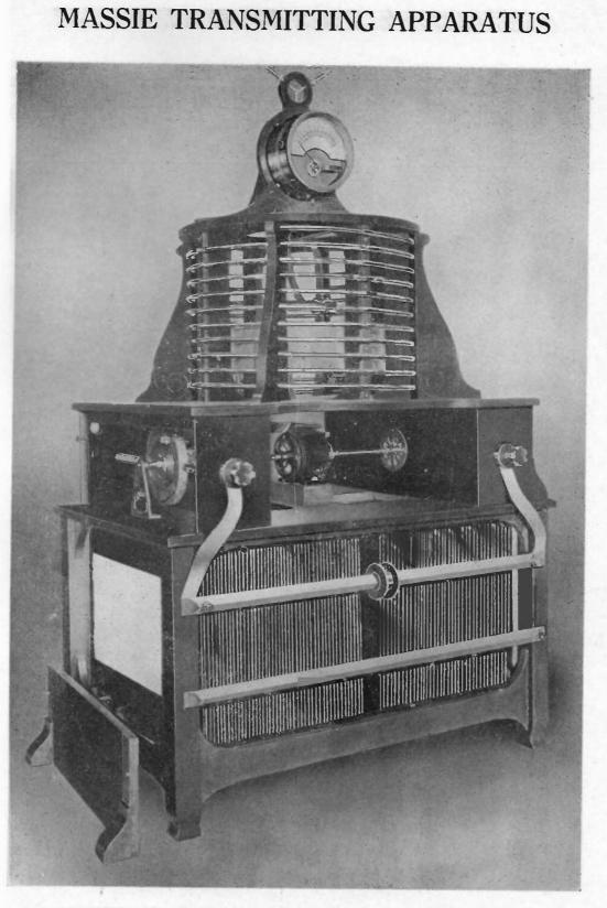
HELIX, PLATE CONDENSER, HOT WIRE AMMETER AND ANCHOR GAP
