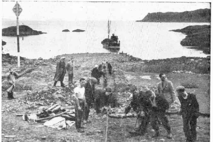
Oban, Scotland: the U.K. end of the cable being pulled ashore by the s.s. 'Glenaray'
