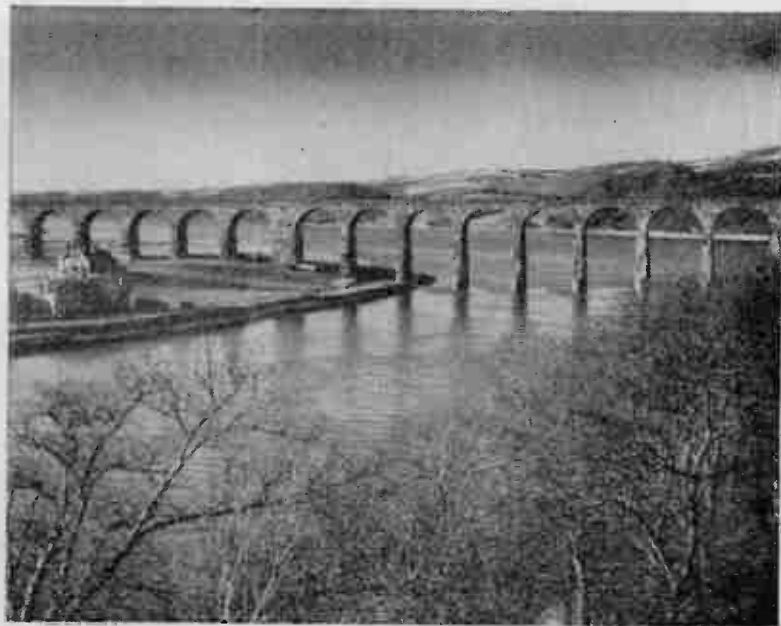
The Royal Border Bridge at Berwick was built by Robert Stephenson more than 100 years ago to carry the railway across the Tweed into Scotland
