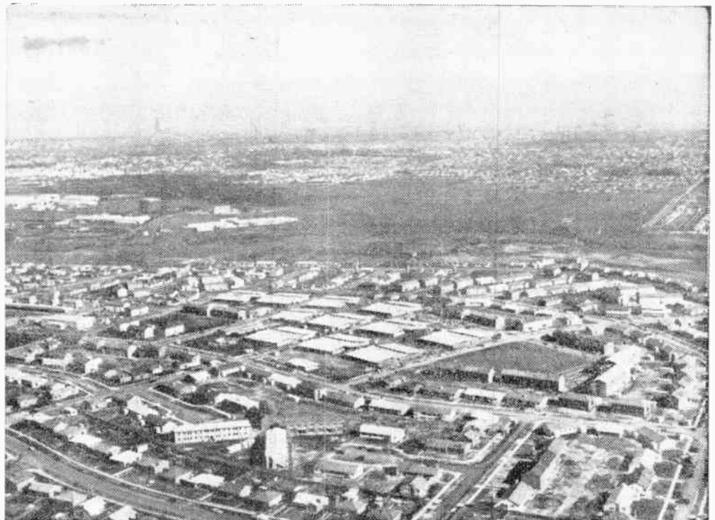
A general view of the village, which covers 117 acres and consists of more than 750 buildings
