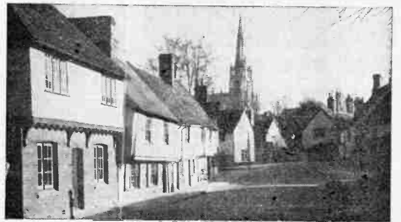
The steeple of St. Mary the Virgin rising above the rooftops of Saffron Walden: on Christmas Eve its twelve bells will ring out over the cold valley
