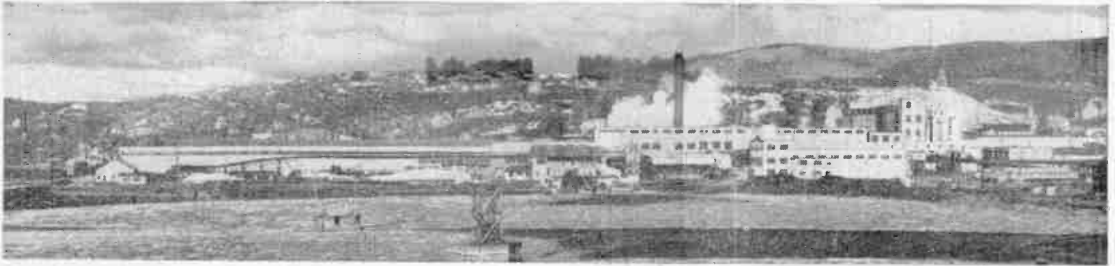
The Bowater paper-mill at Corner Brook is one of the largest in the world: in the foreground are hundreds of thousands of logs waiting to be pulped for newsprint
