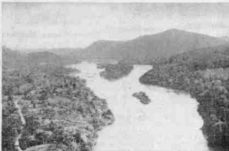
The site of the proposed dam at Ajena, Gold Coast, looking upstream
