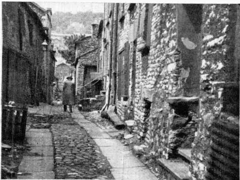
Even today the old buildings of the town with their narrow windows and their unusual arrangement of courts and yards are a reminder of a more turbulent past
