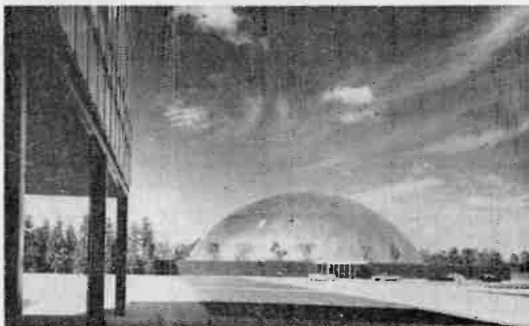
An aluminium-and-steel dome 188 feet in diameter spanning the width of the styling auditorium at the General Motors Technical Centre seen below
