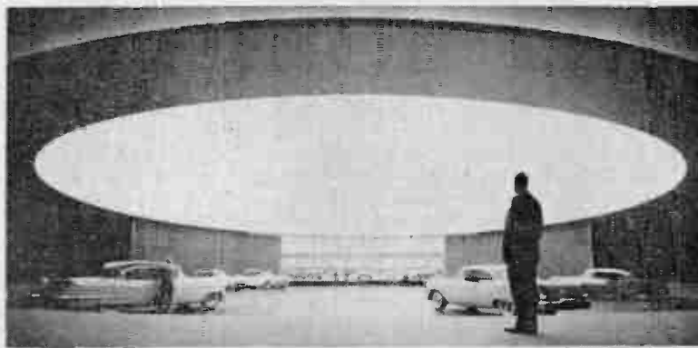
An aluminium-and-steel dome 188 feet in diameter spanning the width of the styling auditorium at the General Motors Technical Centre seen below
