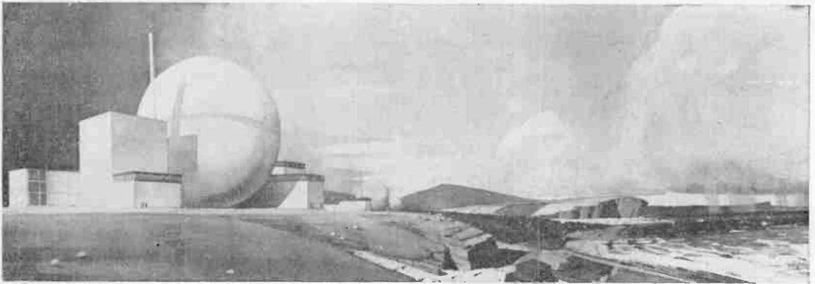
Dounreay, Scotland: what the atomic power-station of the future will look like. The spheres are of steel, 135 feet high, and will house the reactors
