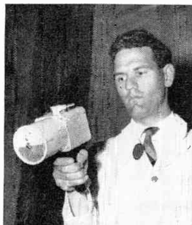
A handy monitor used in testing for areas of suspected radiation
