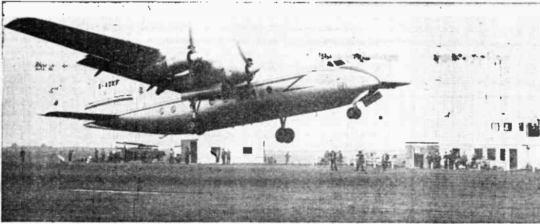
The Handley Page Herald airliner, carrying forty-four passengers, is designed to land on short runways
