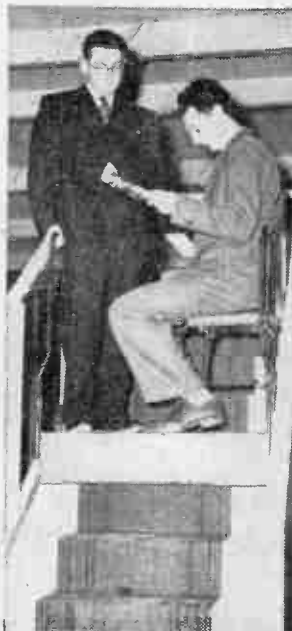
Useful in any house with an invalid—a lift, driven by an electric motor, which runs on rails laid over the stairs
