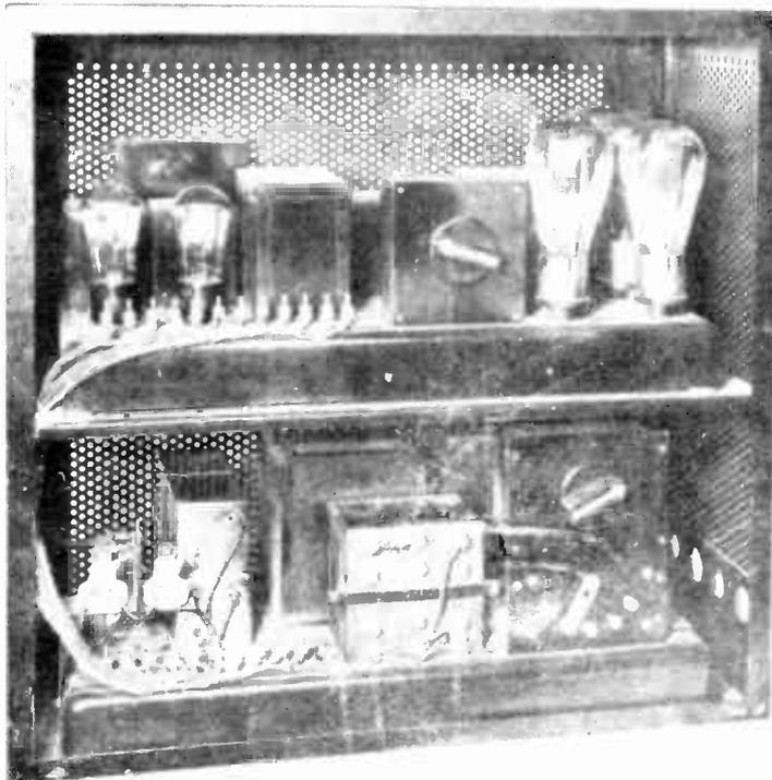
BOTH THE VOLTAGE AND POWER AMPLIFIERS IN THIS EQUIPMENT ARE BUILT INTO A SINGLE UNIT LOCATED IN THE UPPER COMPARTMENT. TWO UX-112A TUBES (LEFT) AND FOUR UX-200 TUBES (RIGHT) ARE IN PUSH-PULL ARRANGEMENT.
