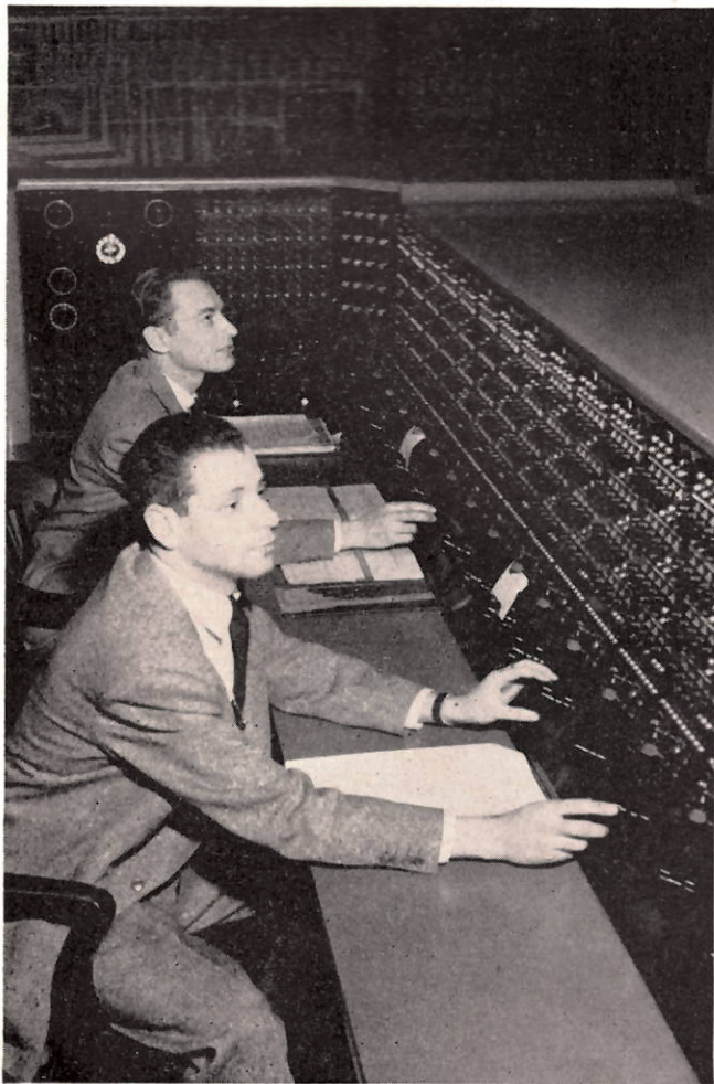
Figure 11 — VOA master-control in New York City. Twenty programs can be handled simultaneously.
