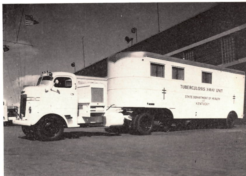
Figure 5—Self-contained, trailer-mounted chest survey unit.
