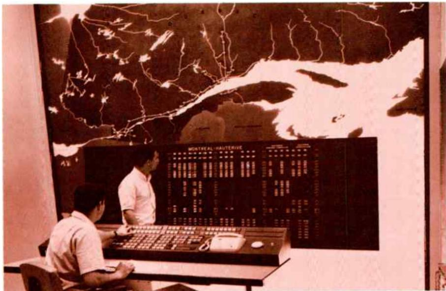
*Figure 4. Electroluminescent map of Montreal-Hauterive power transmission network.*
