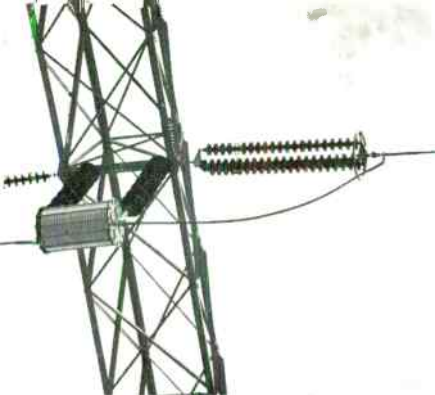
Figure 8. Very elaborate coupling capacitor (right) and frequency trap (above) is required for power lines. Cost may exceed that of a high capacity microwave terminal, particularly on very high voltage lines.
