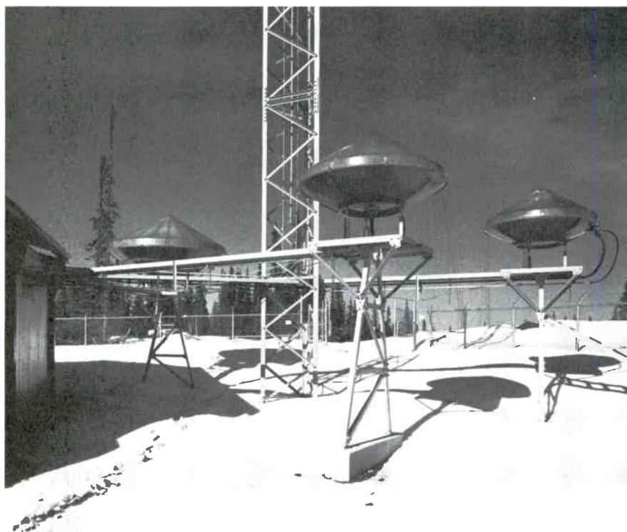
Figure 10. Radomes are sometimes used to protect antennas from weather and debris. The problem is particularly severe where reflectors are mounted horizontally, illuminating a passive reflector which redirects the beam horizontally to a distant site.
