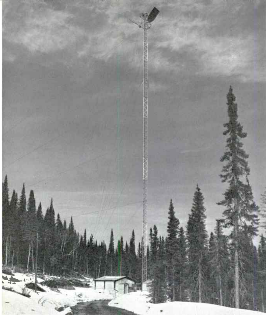
Figure 1. A “periscope” antenna system can provide path clearance without the expense and transmission impairments of a long section of waveguide.
