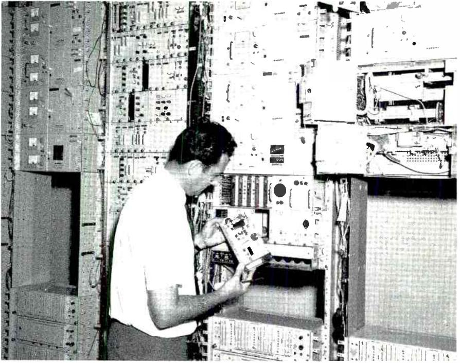
*Figure 5. Lenkurt 76 microwave radio system provides updated communications capabilities at White Sands Missile Range. To left of radio is 57B path protection system.*
