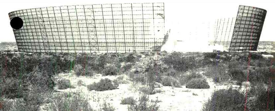
*Figure 1. Radar is first range instrument to "see" missile. Installation at White Sands Missile Range is surrounded by clutter shield.*
