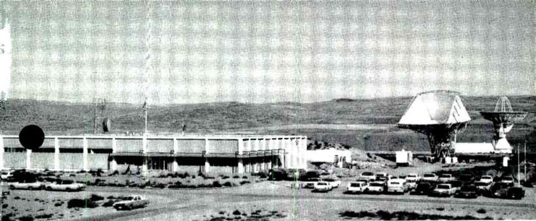
*Figure 1. Brewster Flat ground station, with folded-horn and Cassagrain antenna (right, in distance). Microwave antennas are visible above building.*
