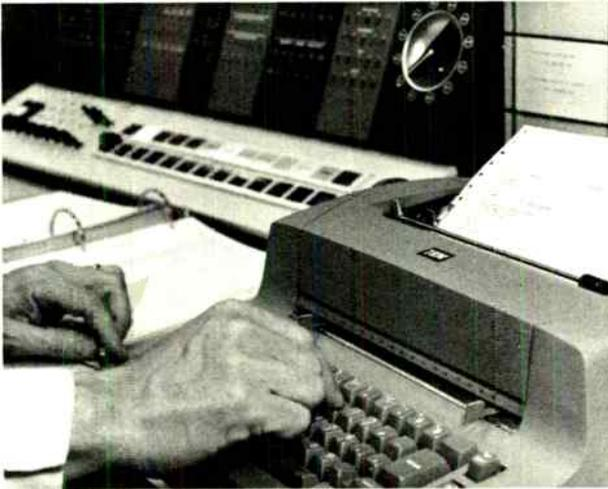
*Figure 3. Electric typewriter allows engineer to supply data to computer as design problem progresses. Results of computation also appear on the typewriter.*
