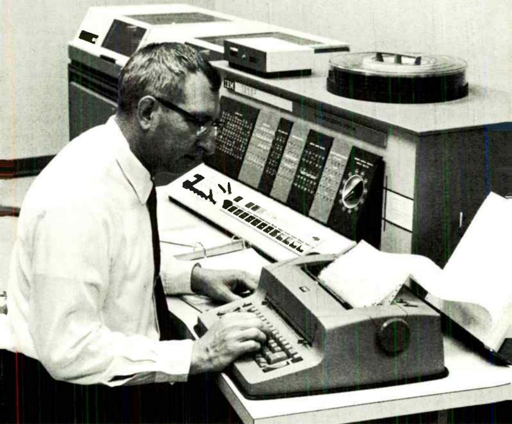
*Figure 1. Typical scientific computer is the IBM 1620 II, used at Lenkurt. Behind the central processing unit is magnetic disc storage drive.*
