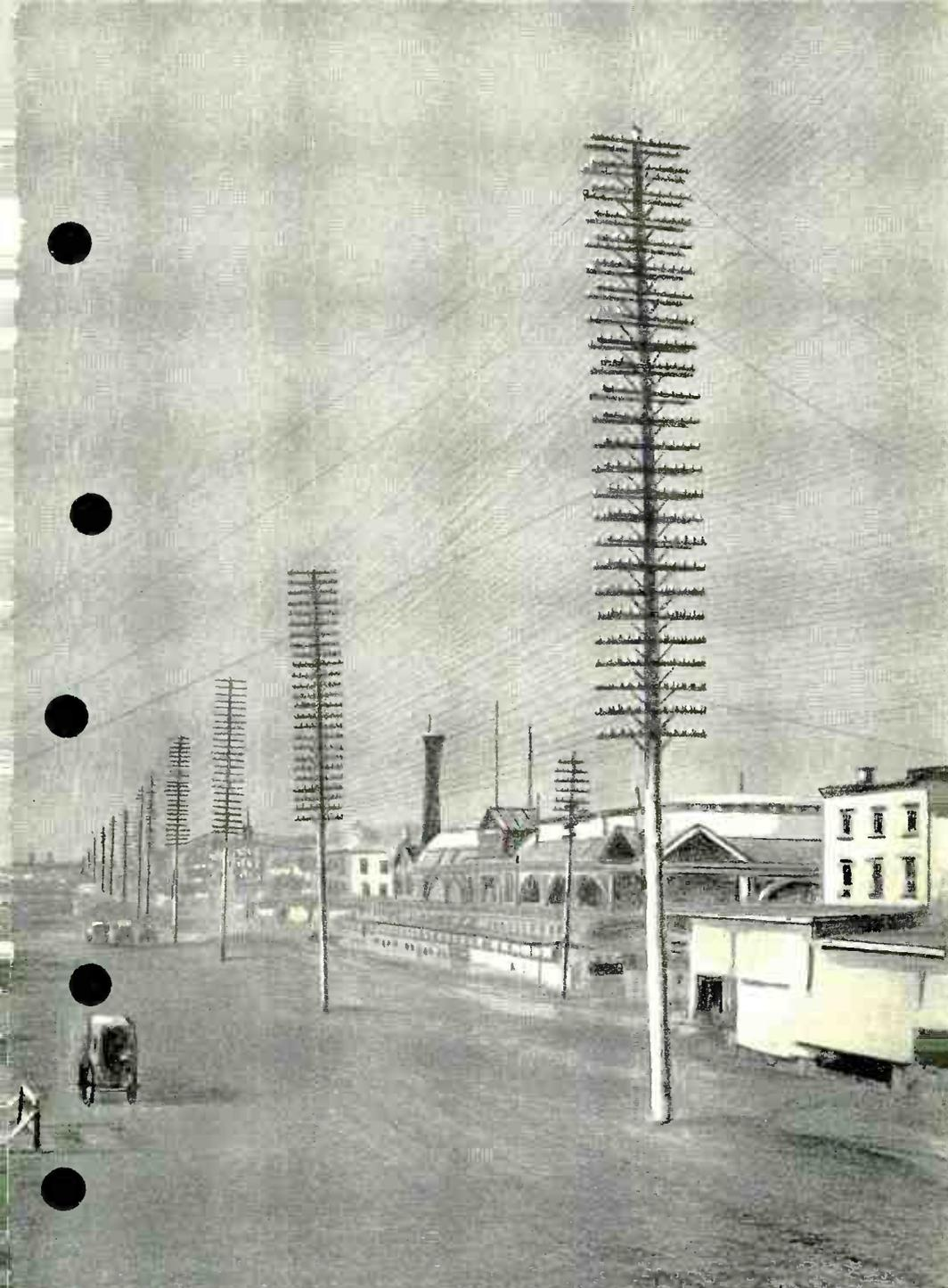
*Figure 4. In the early days of telephony, a pair of wires was needed for each trunk circuit. Often, hundreds of wire pairs had to be strung up on a single pole line to provide the necessary number of trunk circuits between metropolitan areas.*
